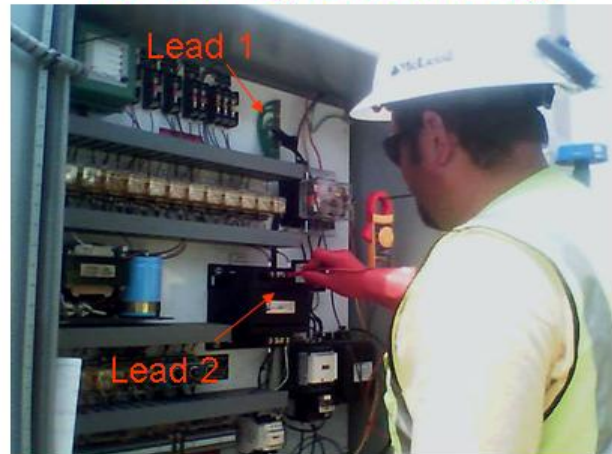
Correct way to read voltage
